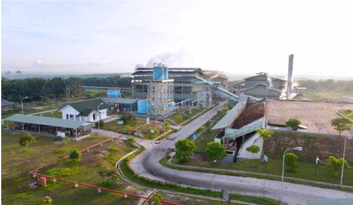
Pabrik Kelapa Sawit PT Borneo Indah Marjaya, Kalimantan Timur CPO Mill of PT Borneo Indah Marjaya, East Kalimantan
